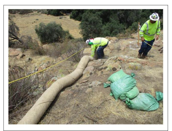
**Photo 6:** Crews were observed installing fiber rolls along the downslope side of the site at P 278746 (C 157) for sediment control in accordance with the Erosion Control Plan and SWPPP (MM HYD-1, MM BIO-7, and APM HYD-09). To prevent potential impacts to cultural resources in accordance with the HPMP (MM CUL-1), gravel bags were used to secure the fiber rolls to the ground surface instead of shoveling a shallow trench and then pounding in wooden stakes.
